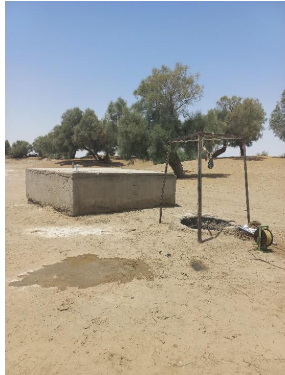
Dug well at TW1– Thul
