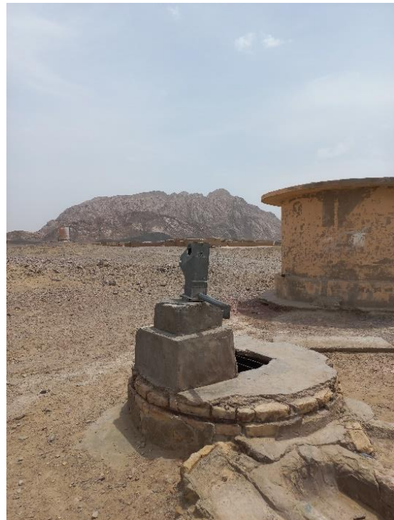
Dug well at W4 – Humai
