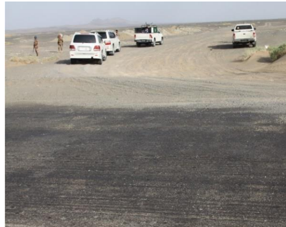
View of the Access Road to the Reko Diq from N-40 Highway
