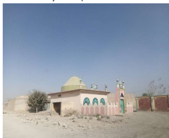
Mosque at Spezand settlement
