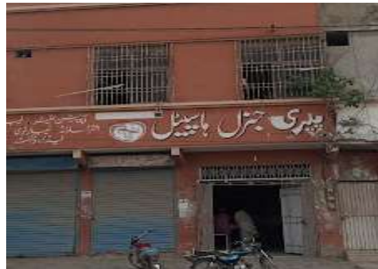
General Hospital in Pipri Settlement
