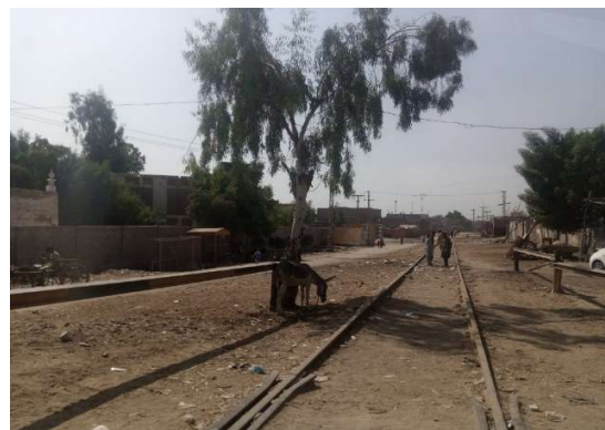
Railway Track near Dadu
