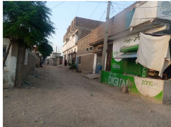
Un-sealed road at Larkana
