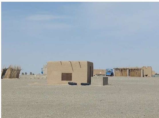
Kutcha House at Rajai Settlement
