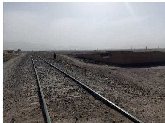
Railway Track near Spezand
