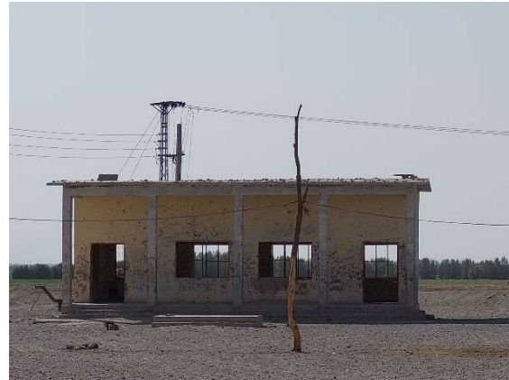
Primary School at Tahlab Settlement
