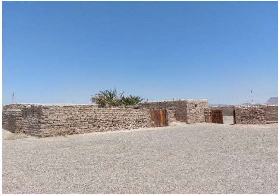
Kutcha House at Tahlab Settlement
