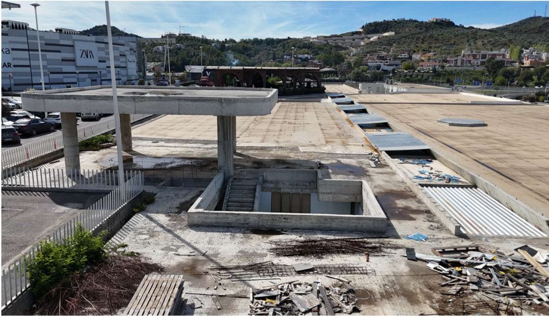
Figure 5-10 Views of the Project Plot from Closest Buildings Source: Eastern Bus Terminal (December 2024)
