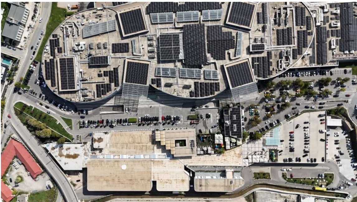
Figure 4-3 Photos from the site
