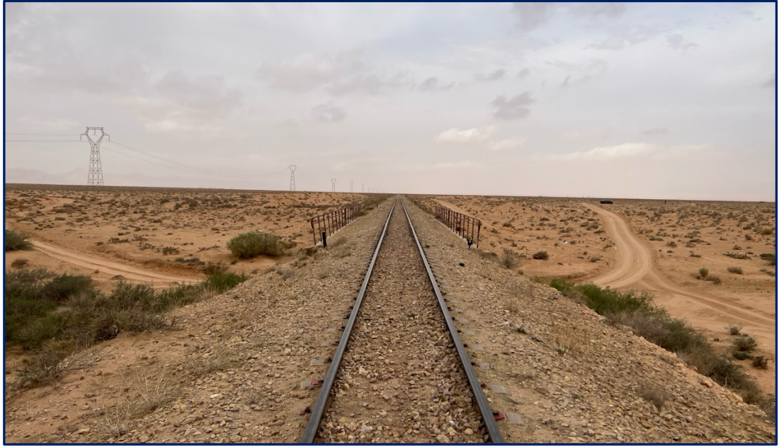
Figure 2.3 - Transmission line Bouchama – Mdhilla (150 kV) and railway located south of the solar PV plant
