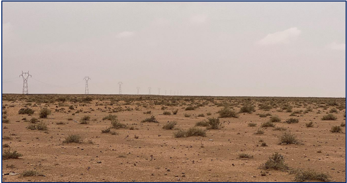
Figure 2.3 - Photo of the 150 kV transmission line in the Southern sector of the solar PV plant
