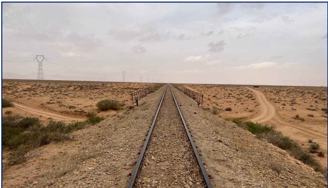
Figure 2.5 - Transmission line Bouchama – Mdhilla (150 kV) and railway located south of the solar PV plant
