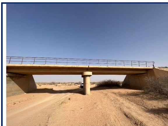
Figure 7.10 - Bridge with two spans, each with a 11.6 m span
