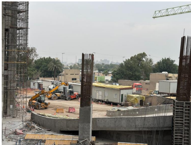
Passenger Car exit ramp
