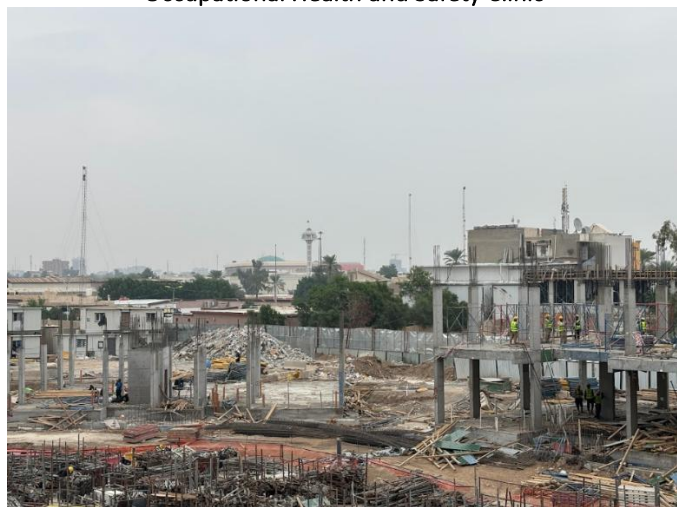
Ongoing villa construction work
