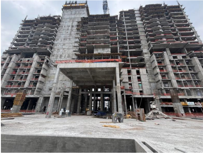
Ongoing Construction work
