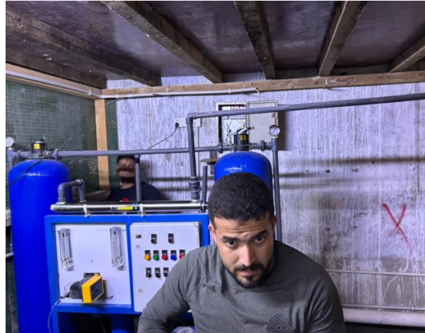
RO Maintenance work
