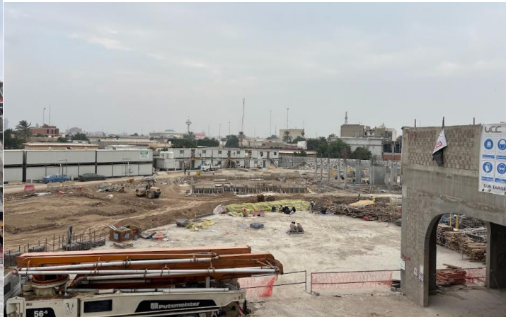
Excavation works ongoing at site
