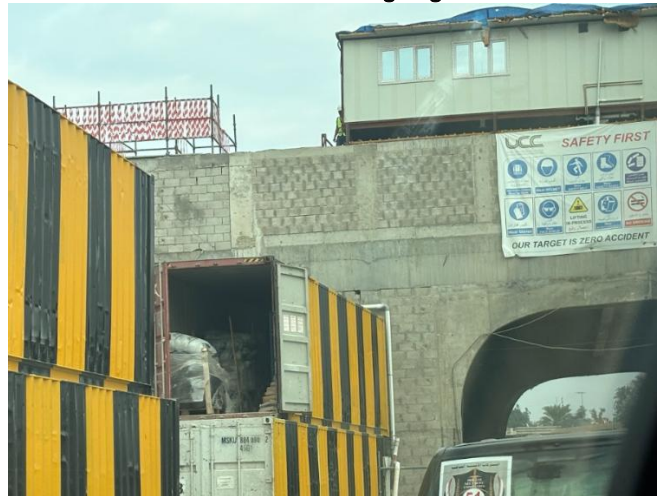
Safety instructions displayed at site
