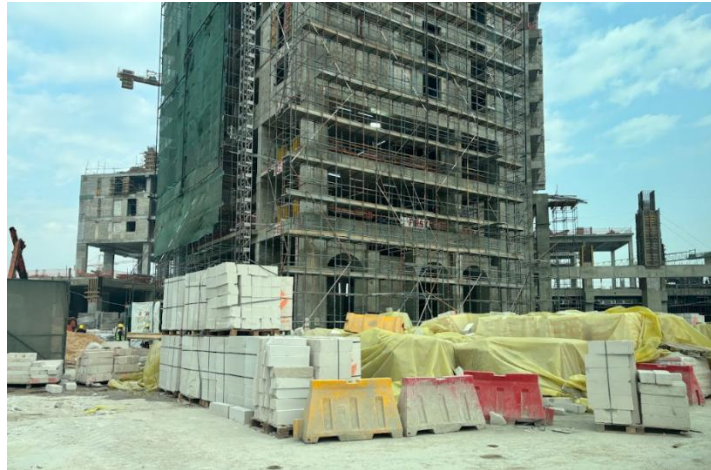
Concrete blocks stored at on-site premises
