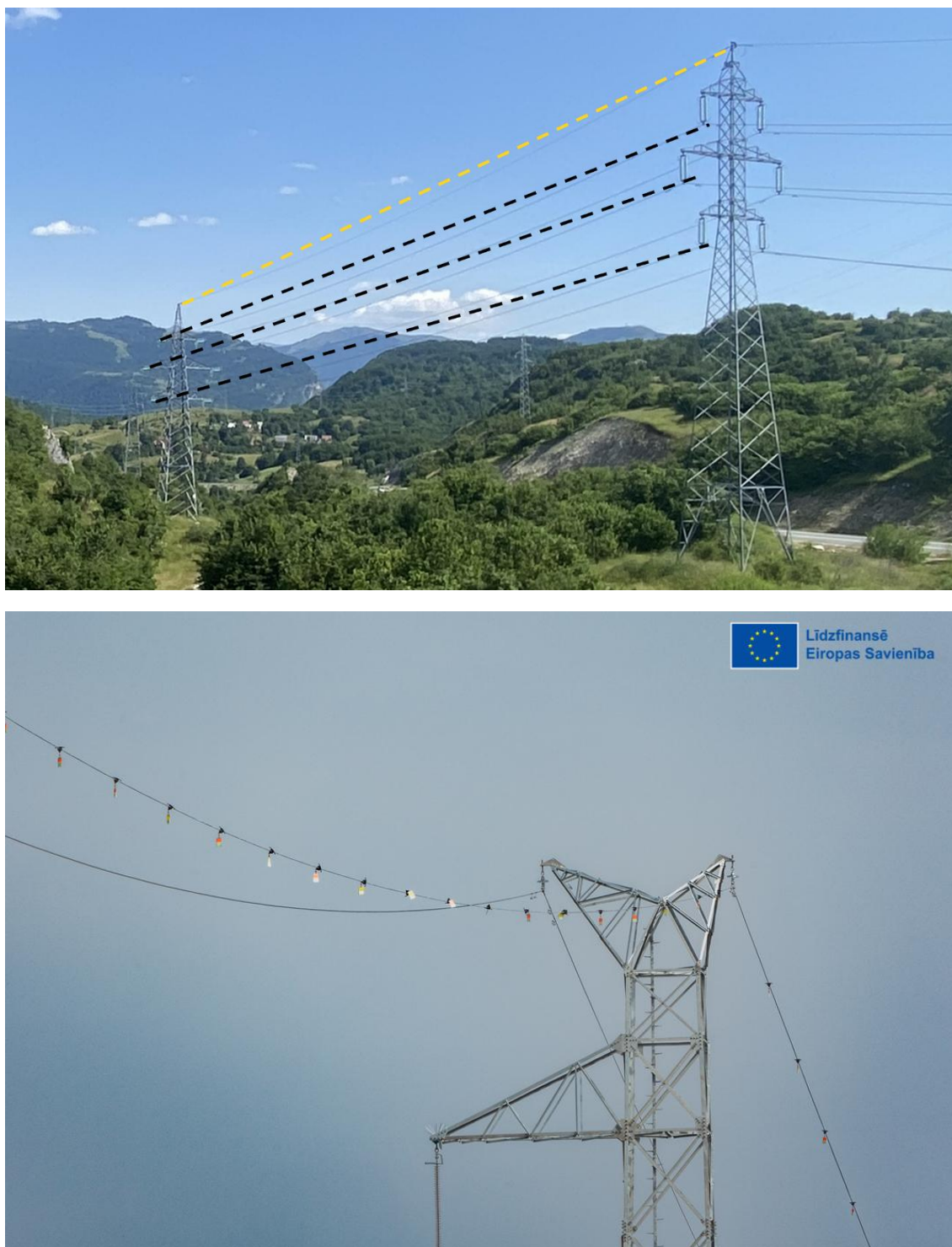
Figure E.3: Example of an OHL provided by Project Proponent with Firefly placement in yellow (top). Installed dynamic diverters on a single 330 kV line (bottom).
