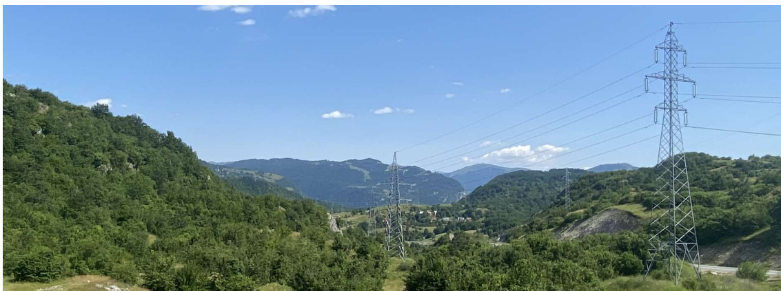
Figure 2.4: Example of an overhead line
