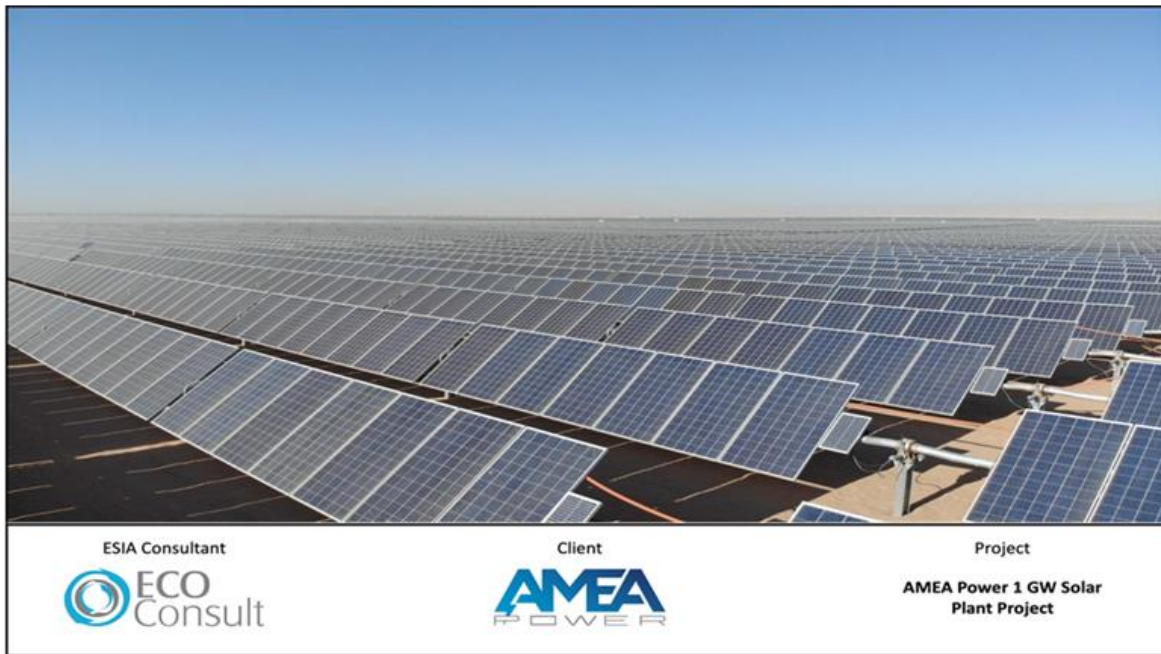
Figure 4: Typical Power Arrays composed of PV Panels
