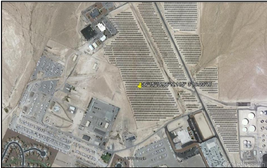
Figure 21: PV Modules Installed near the Nellis Air Force Base in Nevada – USA
