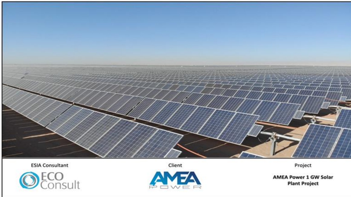
Figure 3: Typical Power Arrays composed of PV Panels
