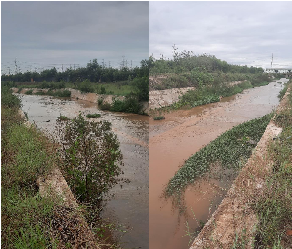
Figure 3-4: Storm/ Public drain bordering the western side of the project site
