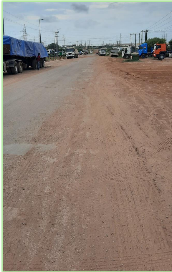
Figure 3-5: Adjoining Road north of proposed project location
