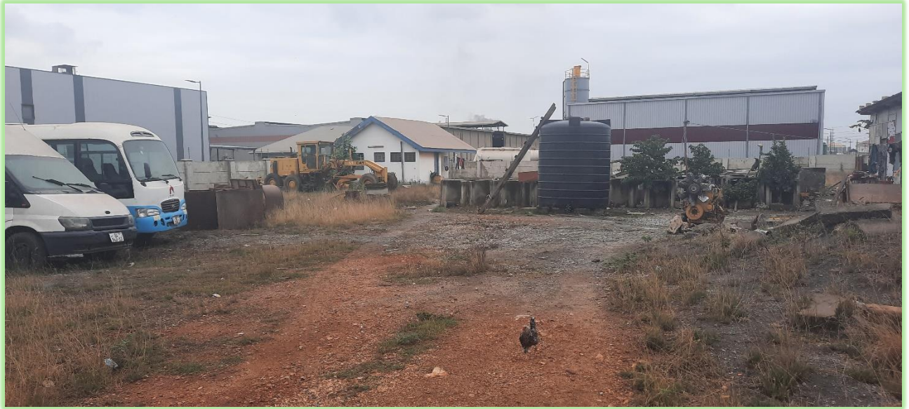
Figure 3-3: Red Sea facility at north-western side of project site
