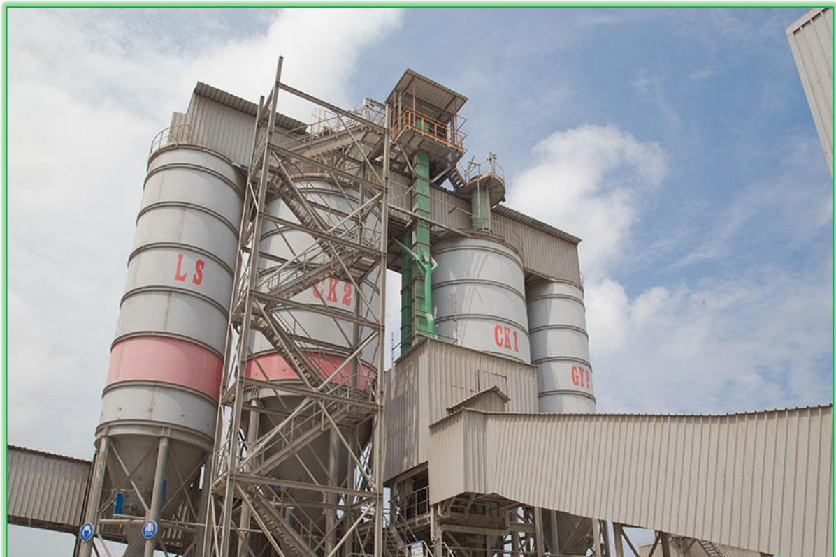
Figure 3-8: Existing raw material silos
