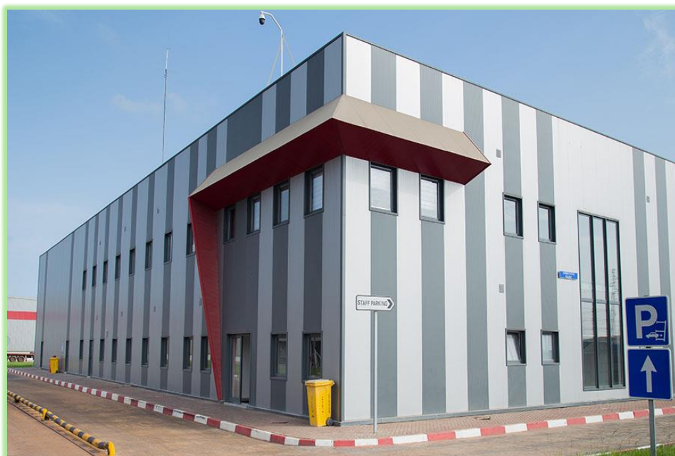
Figure 3-12: CBI Ghana Limited's administrative and technical building
