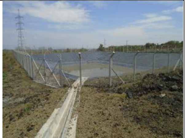
A fenced Brine pond with lining one of the drilling well pad
