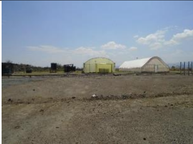
Green houses under preparation within the Menengai well 3 site
