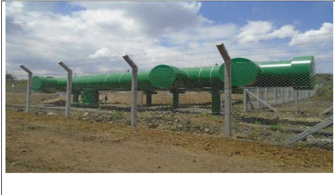
Photo 4-2: OTTL, Globeleq and Sosian steam interphase point with the GDC installed steam gathering system
