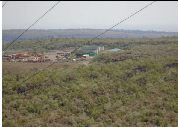
Water storage tanks viewed from Mlima punda.
