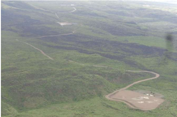
Section of newly done access road and well pads within the caldera as observed from the Menengai view point
