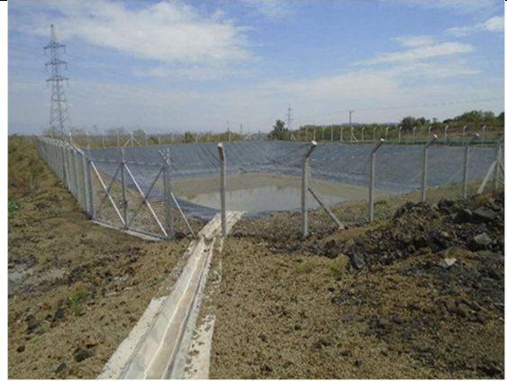
A fenced Brine pond with lining one of the drilling well pad
