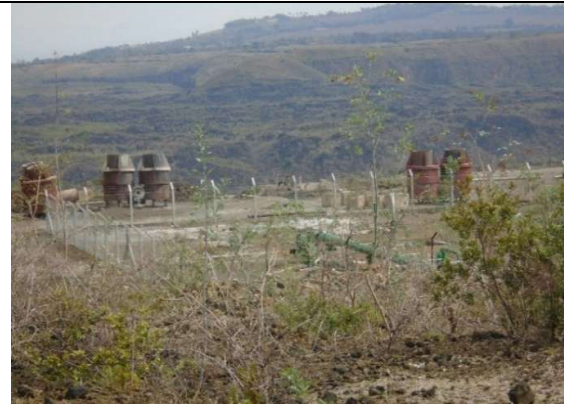
Non functional discharge wells
