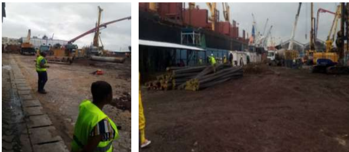
Picture 2 : View of the project site
