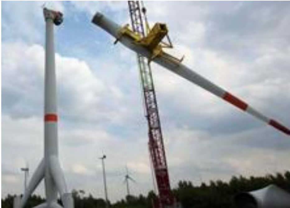
FIGURE 2-8: EXAMPLE OF WIND TURBINE UNDER CONSTRUCTION 5
