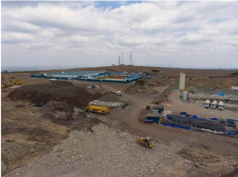
FIGURE 2-6: EXAMPLE OF A GENERAL LAYDOWN AREA AND CONSTRUCTION CAMP
