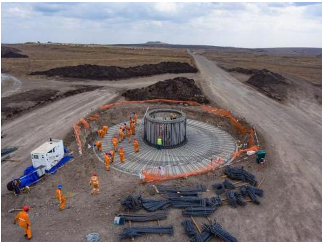
FIGURE 2-7: EXAMPLE OF A FOUNDATION UNDER CONSTRUCTION 4
