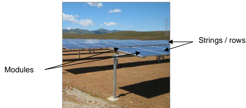
Figure 2.3 Typical layout of panel structures
