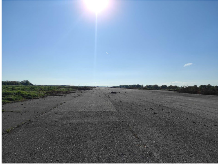
Figure 19: Missing tree and shrub vegetation around the track – May 2023.
