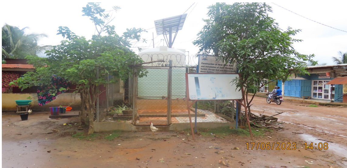
Figure 4-7: A Community Borehole
