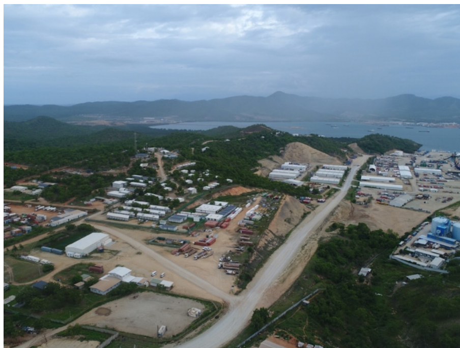
Plate ES2 – The AES Industrial Park
