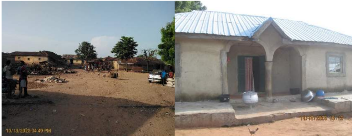
Plate 4.17: Cement block housing Structures observed in the Study Areas
