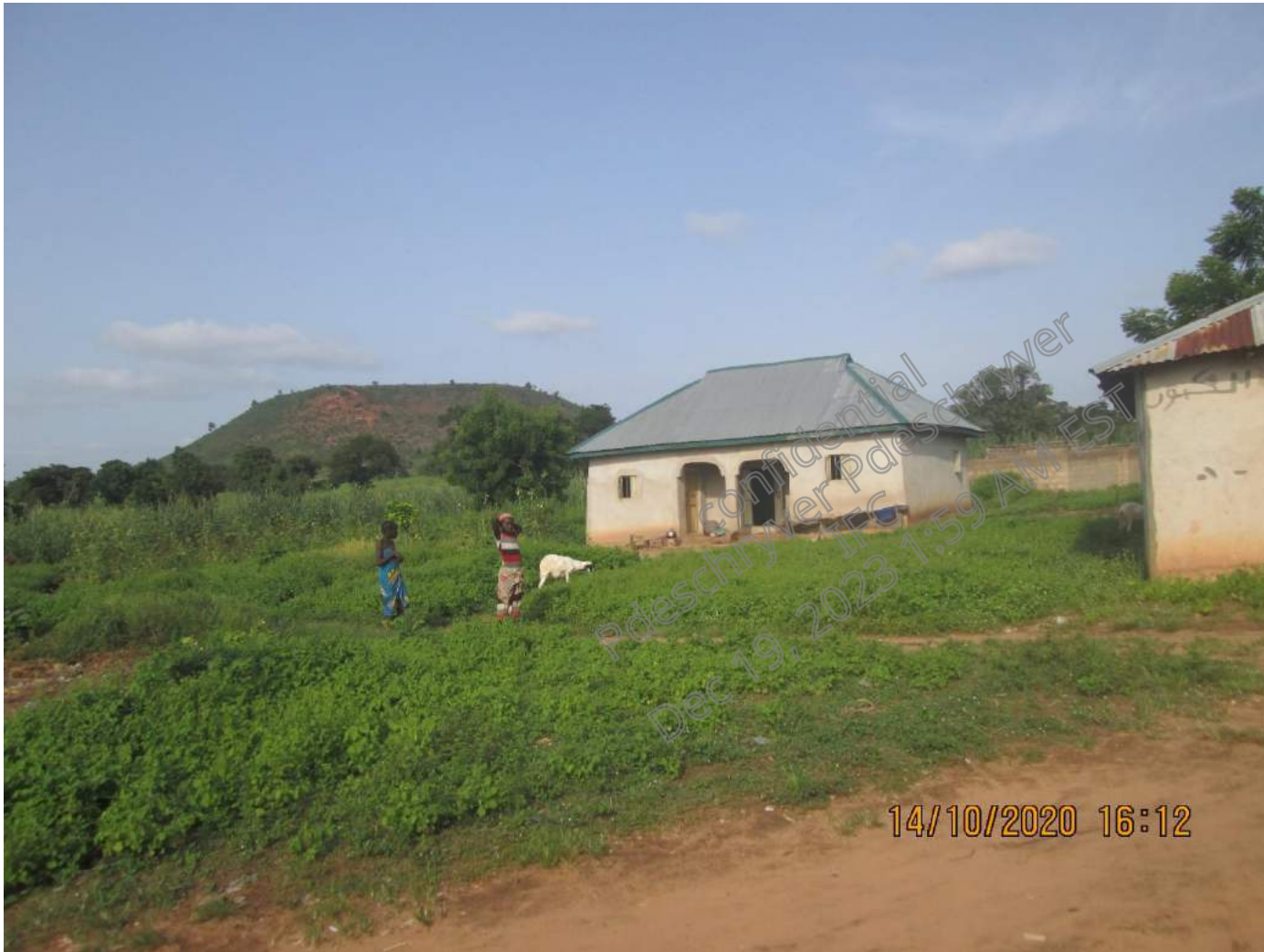
Plate 3.4: Cross sectional image of Kuchitagi community proposed project site
