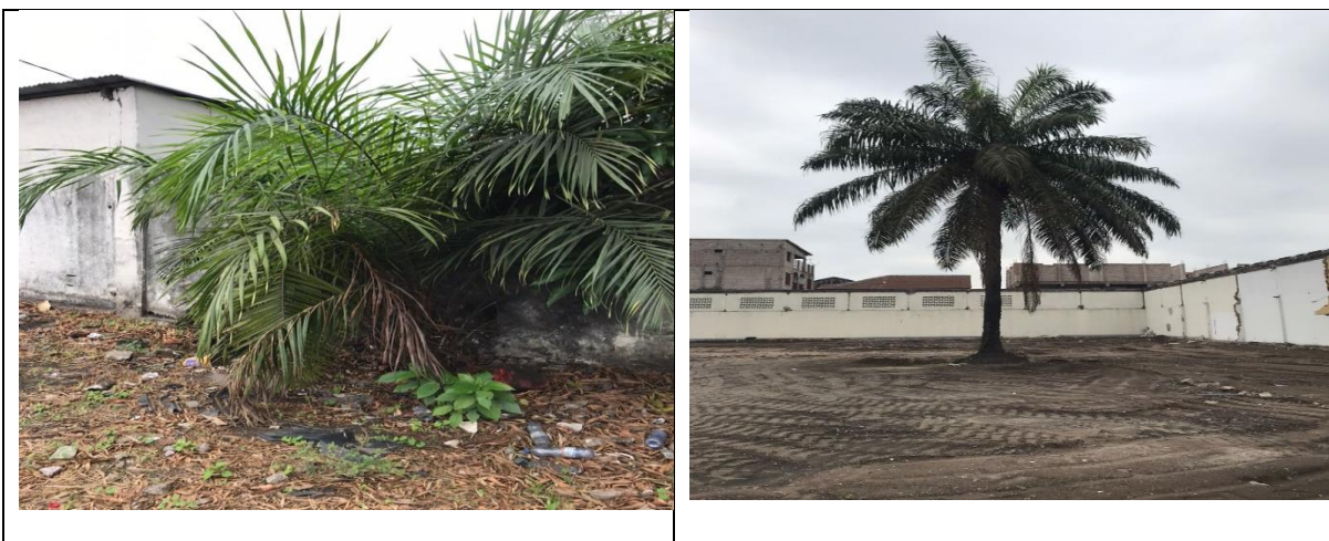
Picture 4. View of palm trees over the Data Center (photo taken 10/21/2022)
