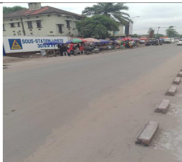
Picture 11. 500m from the site, a SNEL substation
