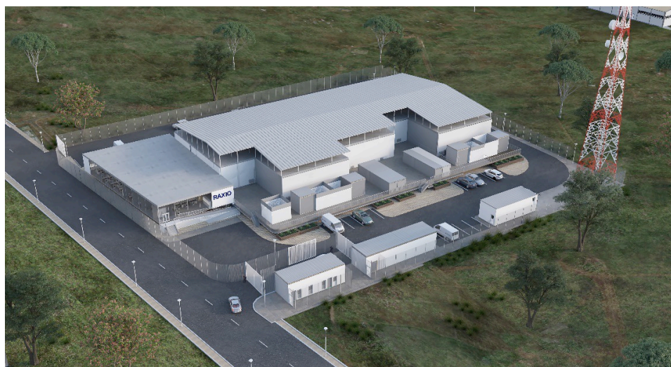
Figure 7: Final view of the construction
