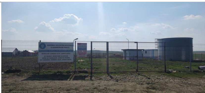
Cragale, Luciu Commune - Sewage treatment plant system
