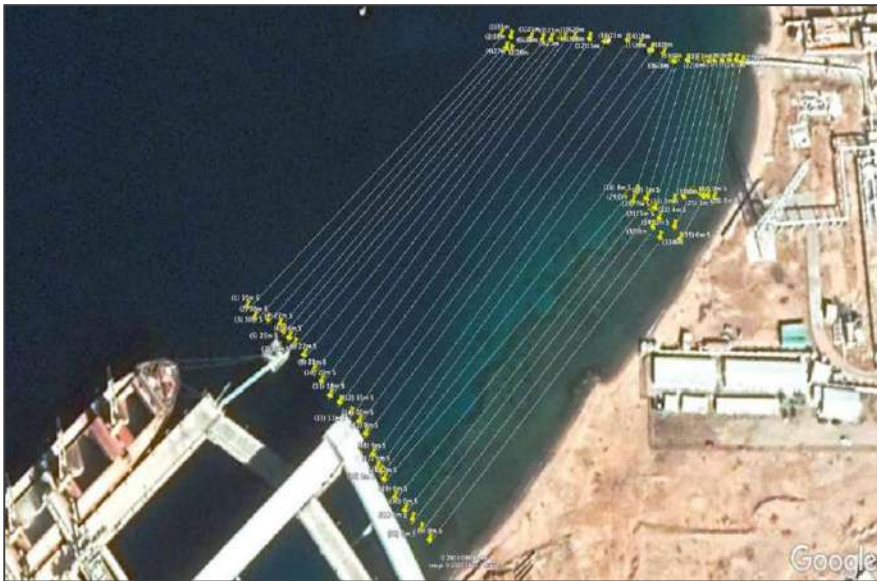
Video Survey at the AAWDC Planned Seawater Intake Area
