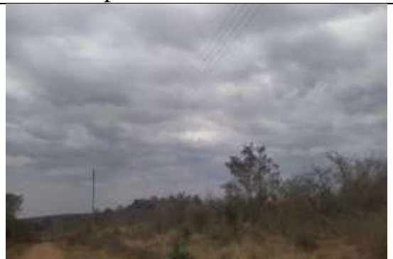
Power line to the project area
