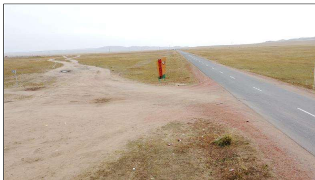
Figure 36. Intersection of the national highway and the main dirt tracks leading to Metagro Farm
