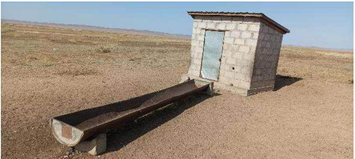
Figure 6-16 - Nagoon well (North)
