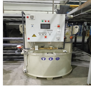
Flocculant preparation and dosing station
