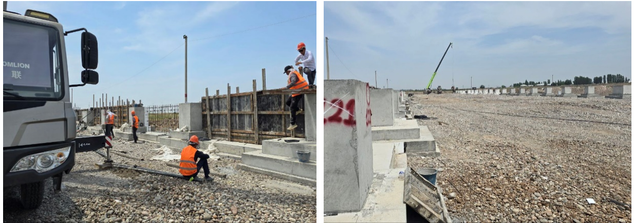
Photo 3: Project zero-cycle construction works (May 2024)
