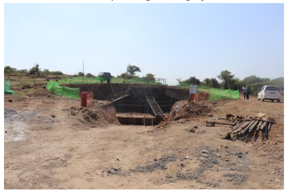
Foundation work at RBR 03 WTG location
