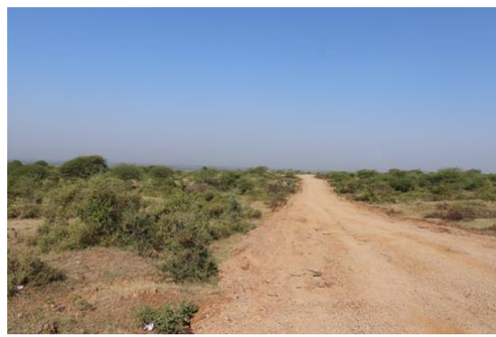
Approach road of RBR
