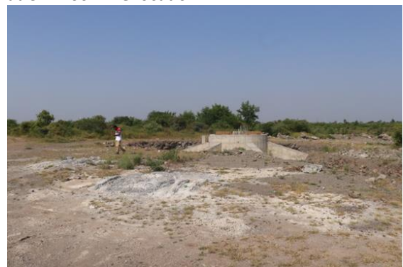
PDV 01 WTG location foundation work
