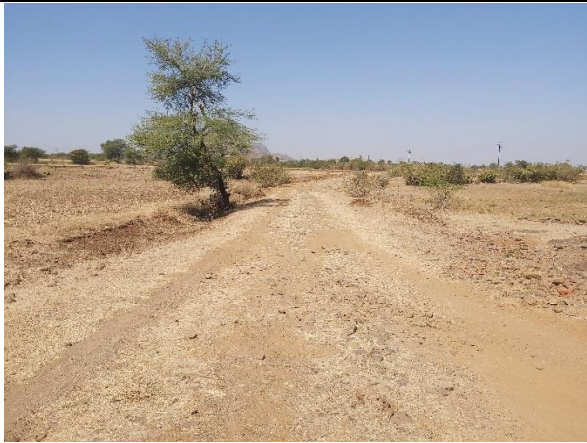
Figure 2-3: View of the existing access road to site
