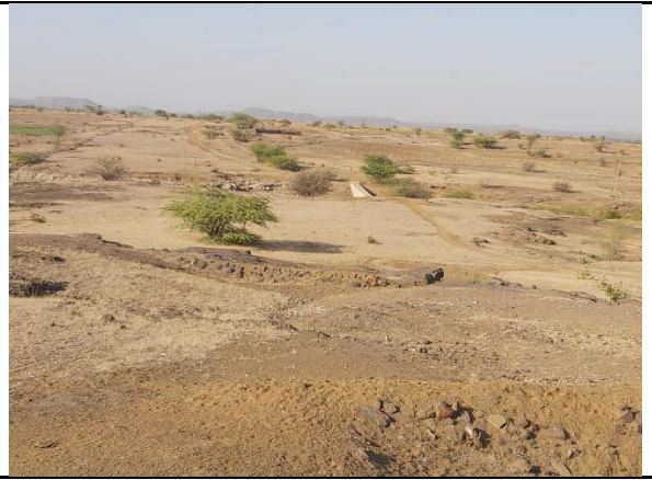
Checkdam adjacent to the Nagpur Plot
