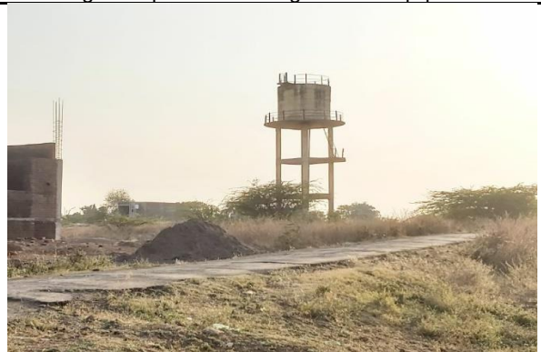
OHT Supplying Drinking water to Nagpur Village
