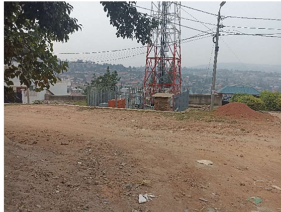
Figure 6.12 Electricity Transmission Masts
