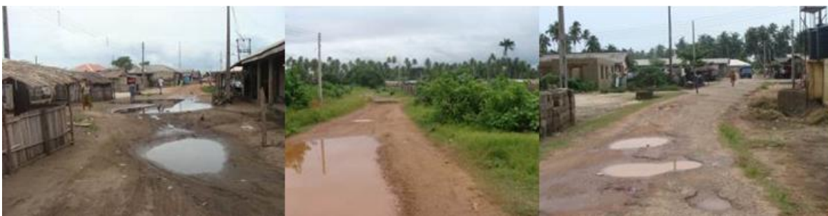
Plate 4.25: Untarred Roads within the LFZ Project Area
