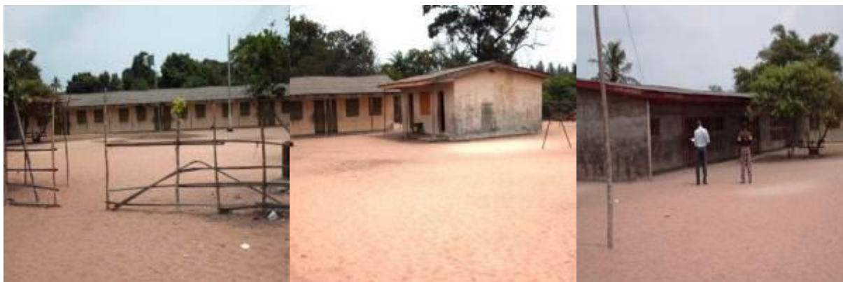
Plate 4.21: Primary School Structures at Idotun, enhanced by USAID/LEAP
