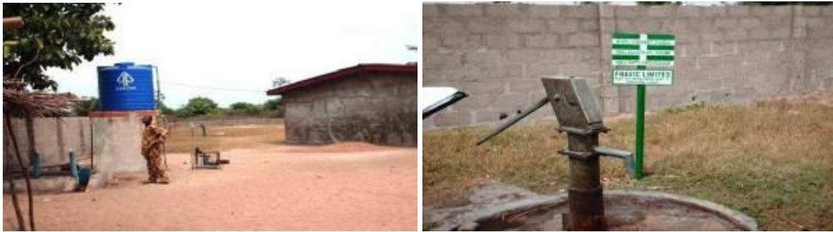
Plate 4.27: A Borehole and Water Tank and Mono-Pump Locate within the Primary School at Idotun, sponsored by USAID and FMOWR, respectively
