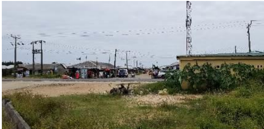
Plate 4.11: Observed Electricity Infrastructure
