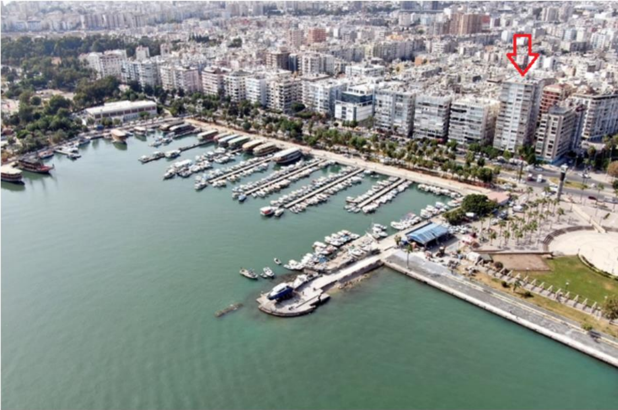
Figure 15: Mentioned high rise building
