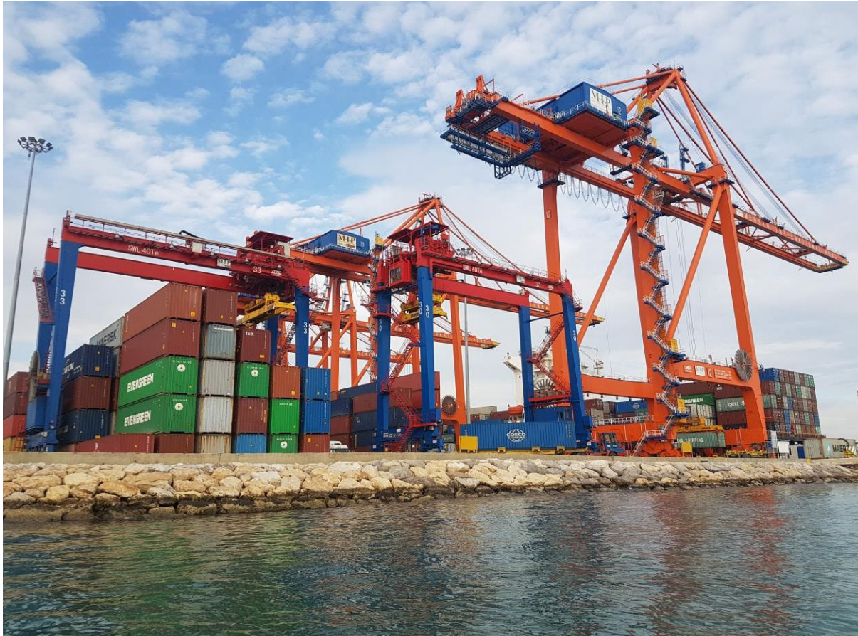
Photo 1. Port and dock structures.
