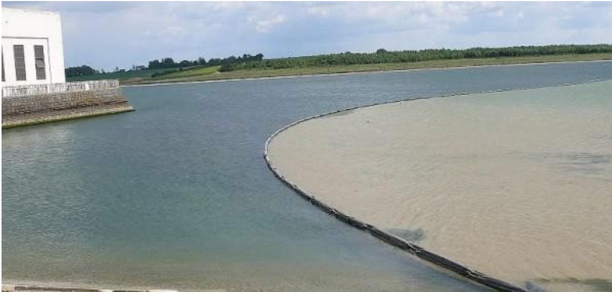
Photo 51. Silt Curtains to Prevent Turbidity
