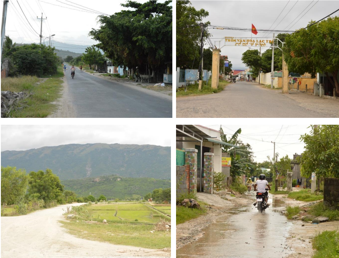
Figure 9.40 A Paved Road in Phu Lac Commune
