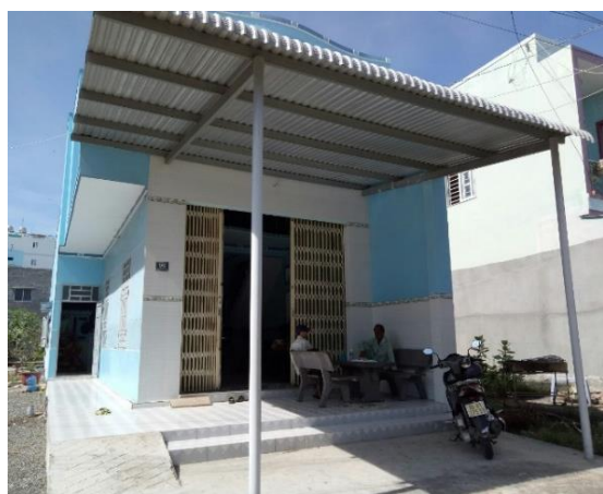
Semi-permanent house in the surveyed area (Lien Huong)
