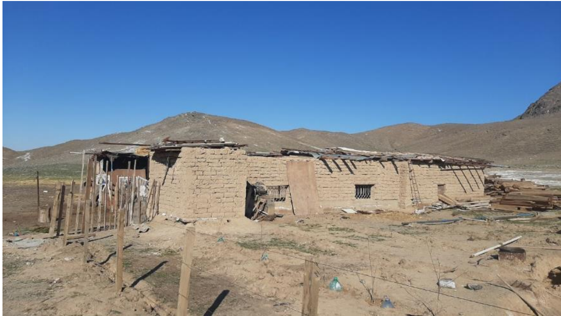
Figure 2-5: Herder Shelter within the Project Area
