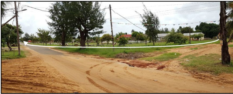
Figure 29: View of the junction of Maritima approach road and tar road. Note overhead telephone and electricity cables.
