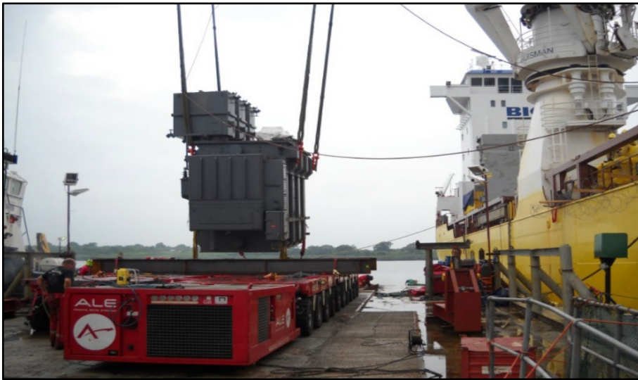
Figure 9: Equipment (Transformer) being loaded directly onto trailers on the barge
