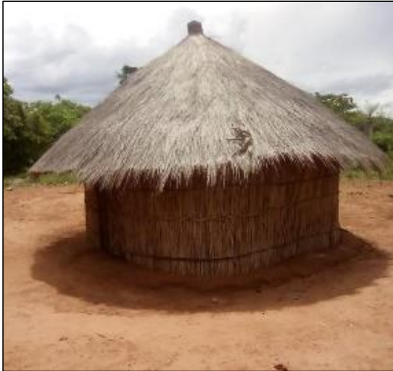
Plate 5 Example of a 'main house' made from reeds with a thatch roof
