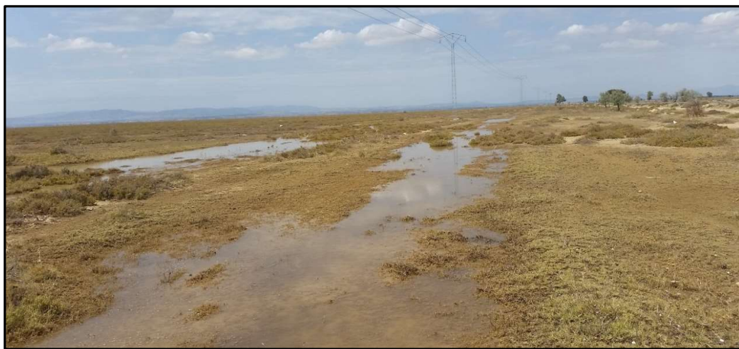
Flooded Area within the Project Site
