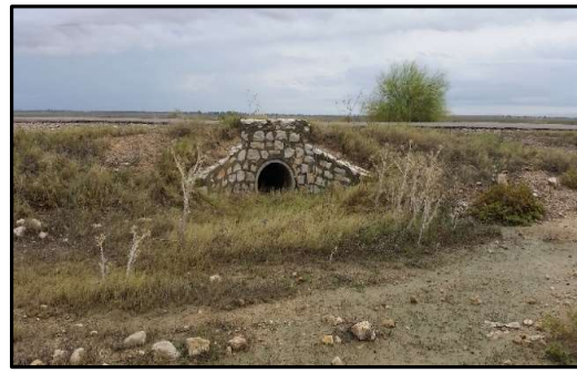
Culvert installed beneath the road along the project site
