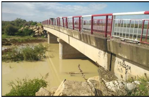
Bridge over Wadi Boughal
