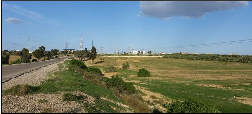
Figure 2.6 - STEG Electrical Substation
