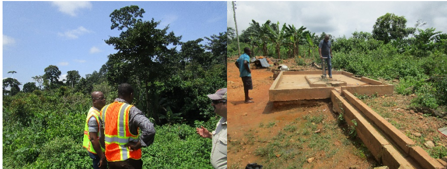
Plate 1-1: Field visit to the project site (Left) and Ohene Nkwanta Community borehole (Right) (SAL 2019)
