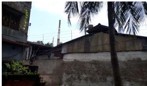
Industry behind the Aruapara STP with Stack
