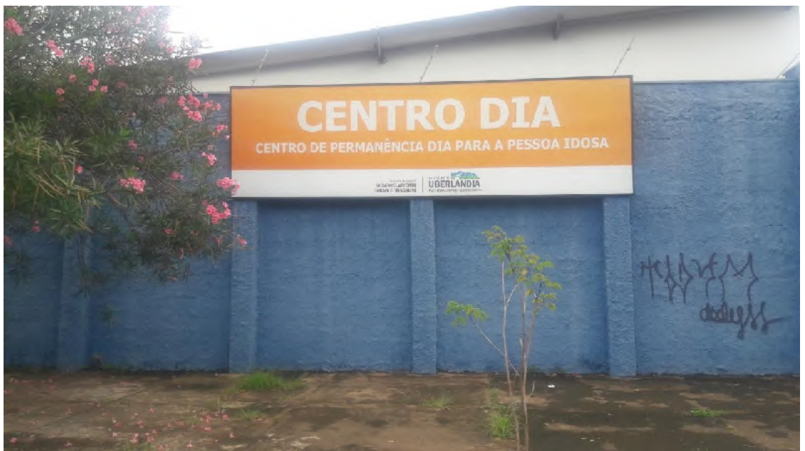
Figure 88 – Centro dia – Day Centre Care for Elderly People in Uberlândia. Source: Pöyry Tecnologia (2018).
