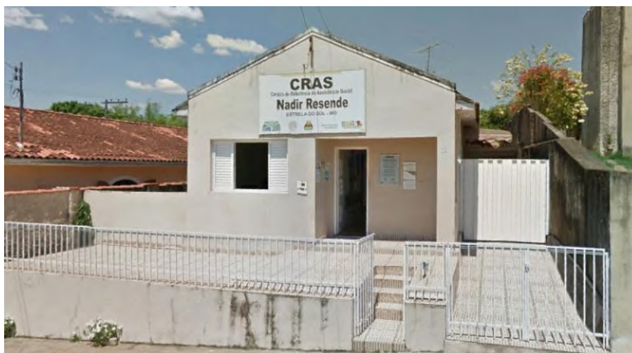
Figure 79 – Social Assistance Reference Centre (CRAS) in Estrela do Sul. Source: Google Earth (2018).
