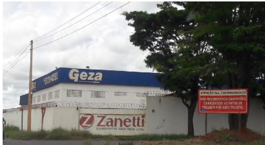
Figure 80 – Geza in Araguari. Source: Pöyry Tecnologia (2018).
