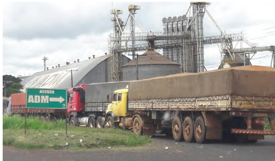
Figure 47 – ADM mill in Araguari. Source: Pöyry Tecnologia (2018).
