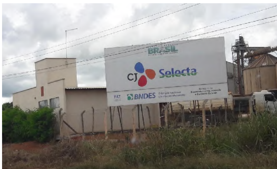
Figure 49 – Selecta mill in Araguari. Source: Pöyry Tecnologia (2018).
