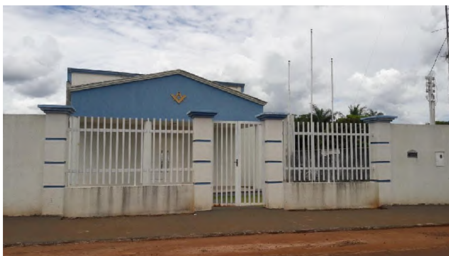
Figure 83 – Indianópolis Masonic Lodge. Source: Pöyry Tecnologia (2018).
