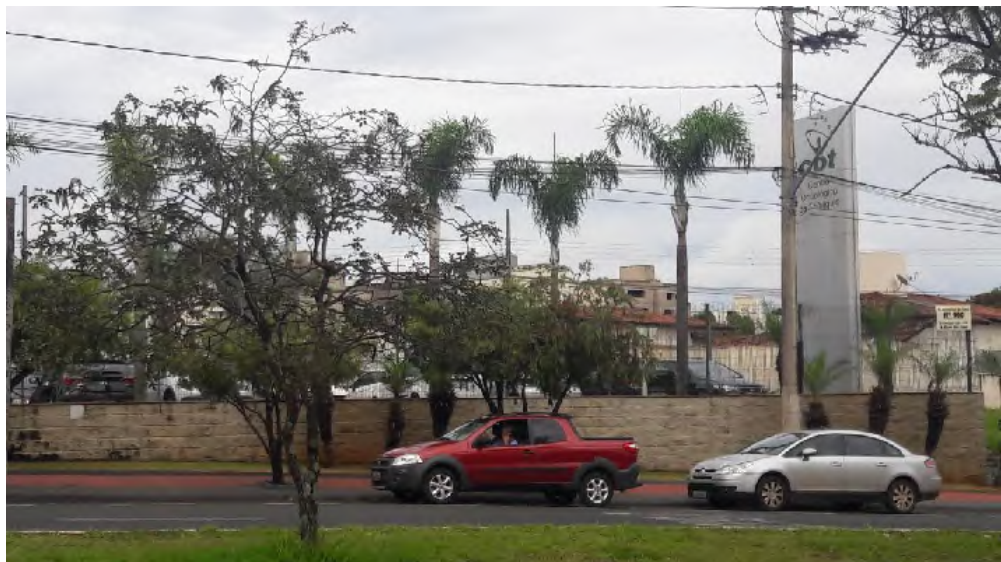
Figure 35 – Triângulo Cancer Centre (COT) in Uberlândia. Source: Pöyry Tecnologia (2018).
