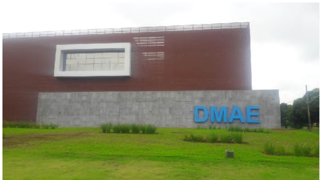
Figure 38 – DMAE office in Uberlândia. Source: Pöyry Tecnologia (2018).
