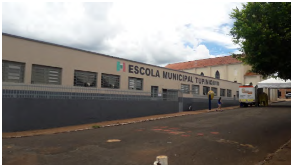
Figure 20 – Tupiniquim Municipal School in Indianópolis. Source: Pöyry Tecnologia (2018).
