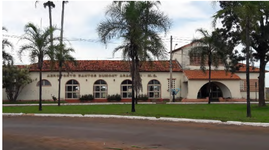
Figure 63 – Airport in Araguari. Source: Pöyry Tecnologia (2018).
