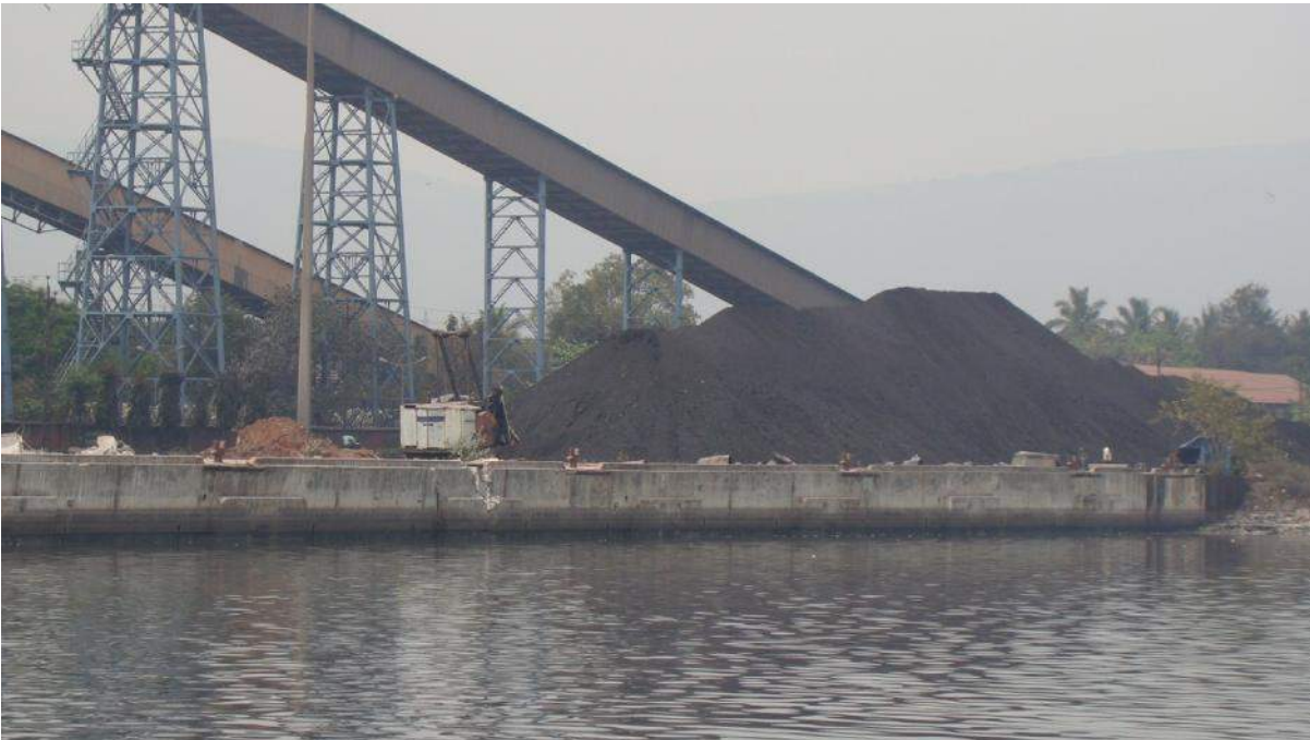
West Q-1 Iron Ore Berth
