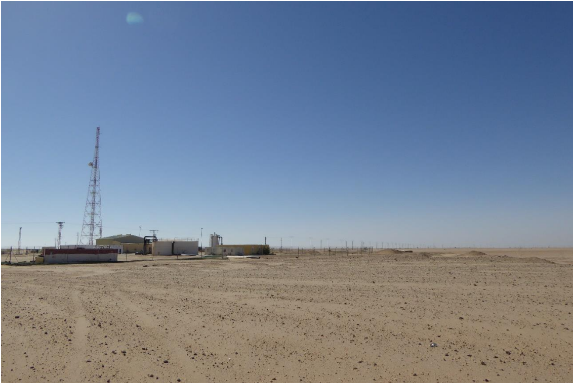
Figure 6: Sondage pumping station
