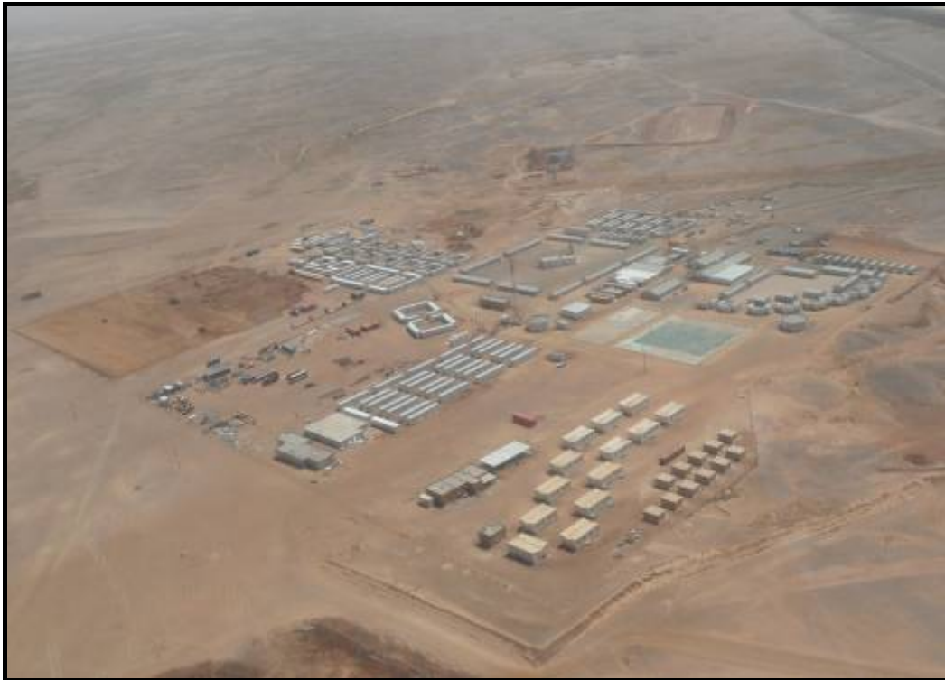
Photograph 3-7: Existing Accommodation Camp
