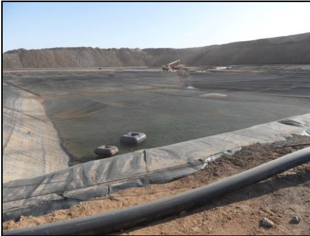
Photograph 3-5: Existing Dump Leach Facility
