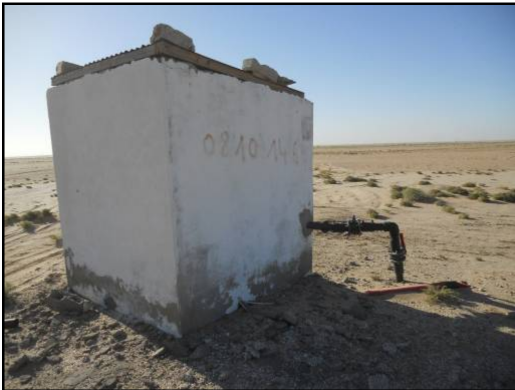
Photograph 3-8: Existing Well at Borefield
