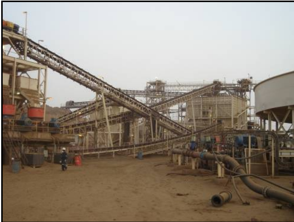
Photograph 3-3: Existing CIL Process Plant
