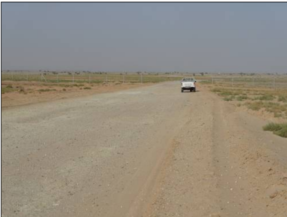
Photograph 3-10: Access Road connecting the Nouakchott–Nouâdhibou N2 highway to the Mine site
