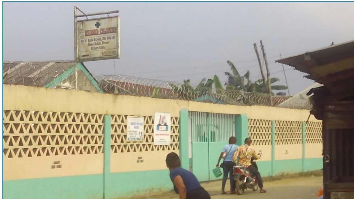
Plate 4.11.1: Health Center at Nchia - Eleme
