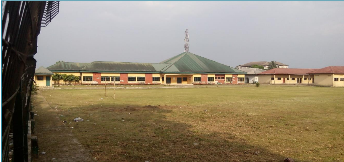
Plate 4.10.5: Comprehensive Secondary School in Alesa – Eleme LGA
