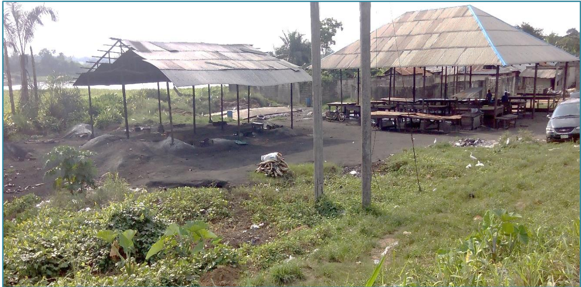
Plate 4.11.2: Abattoir opposite the Aleto (Okulu) River Bridge
