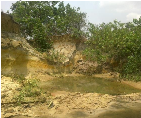
Plate 4.7.3: Collapsed bank of Okulu stream due to sand mining
