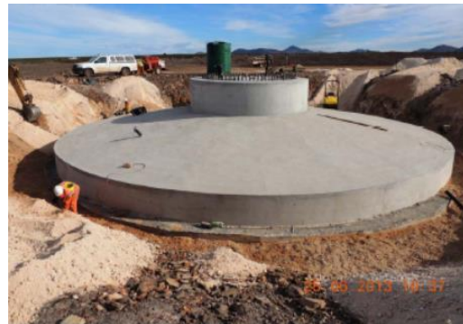
Foundation concrete pour completed and ready for backfilling.
