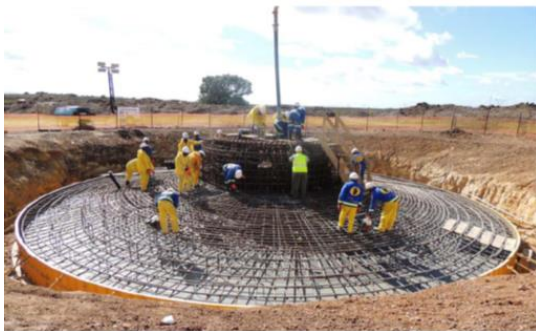
Foundation– Steel fixing stage.
