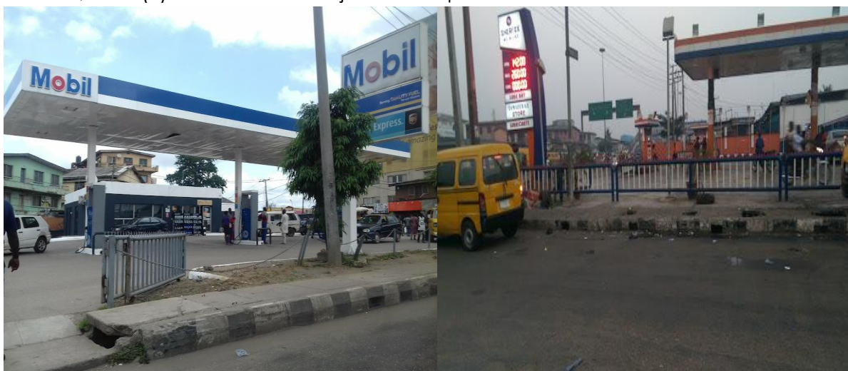
Plate 3.3: Image of Mobil petrol station at Onipanu and Sherfex at Illasamaja. Source: Sustainability Limited, September 2022
