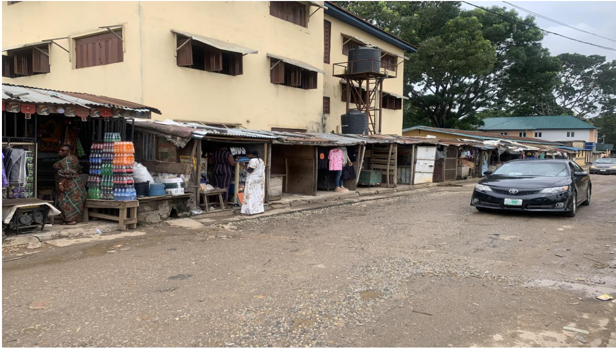
Figure 3- 2: Shows the wooden kiosks and shed at one of the proposed areas for construction. Source: LAMATA, July 2023.
