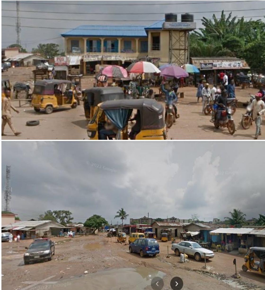
Figure 3- 6: Shows part of the affected structures at the proposed location (Option B) for the Bus Terminal.
